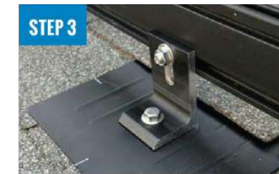
ATTACH L-FOOT TO RAIL
